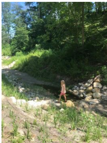
Stone Grade Control Improves Water Quality, Stabilizes the Stream Bed and Bank, and Provides In-Stream Habitat
