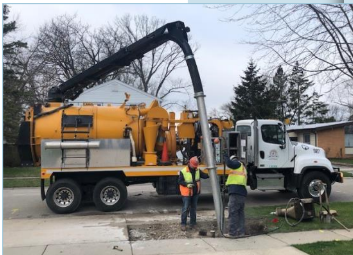
Hydro-Excavator used to repair a water service leak. Village of Wheeling
