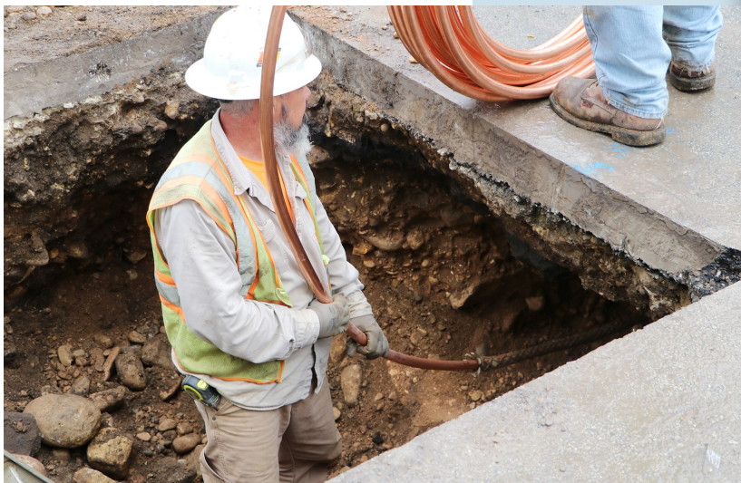
Lead service line replacement
