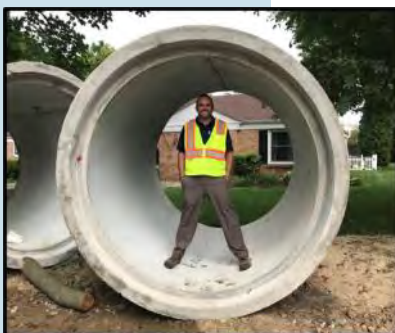
Village Engineer Cooper within an 84" Storm Pipe Along Rockland Road
