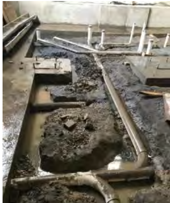
Basement Plumbing for Bathrooms
