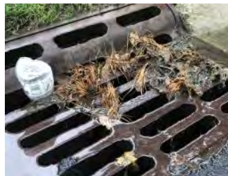
Clogged storm drains prevent water from flowing and draining properly, increasing the chances of ponding water and flooding in neighborhood streets
