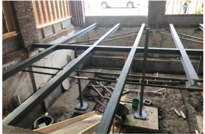
Basement Plumbing & 1st Floor Steel Joists
